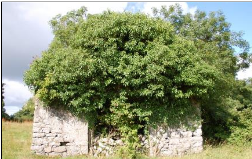
Plate 11-5 East gable with elliptical arch and overgrown dovecote openings above.
